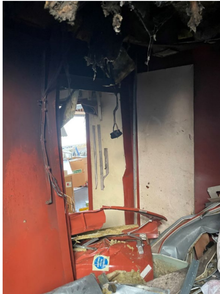
(U) Internal View of Impact Site from Iranian UAV Attack
